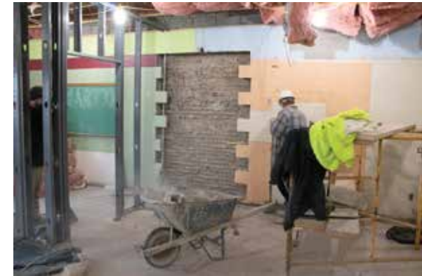
The renovation of Martin Hall begins.
